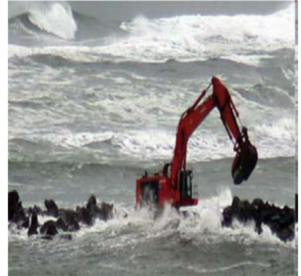
North Jetty Repair / Coos Bay (2002)
